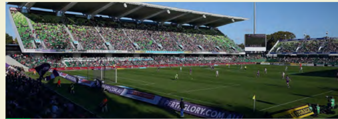
AU Perth Rectangular Stadium
